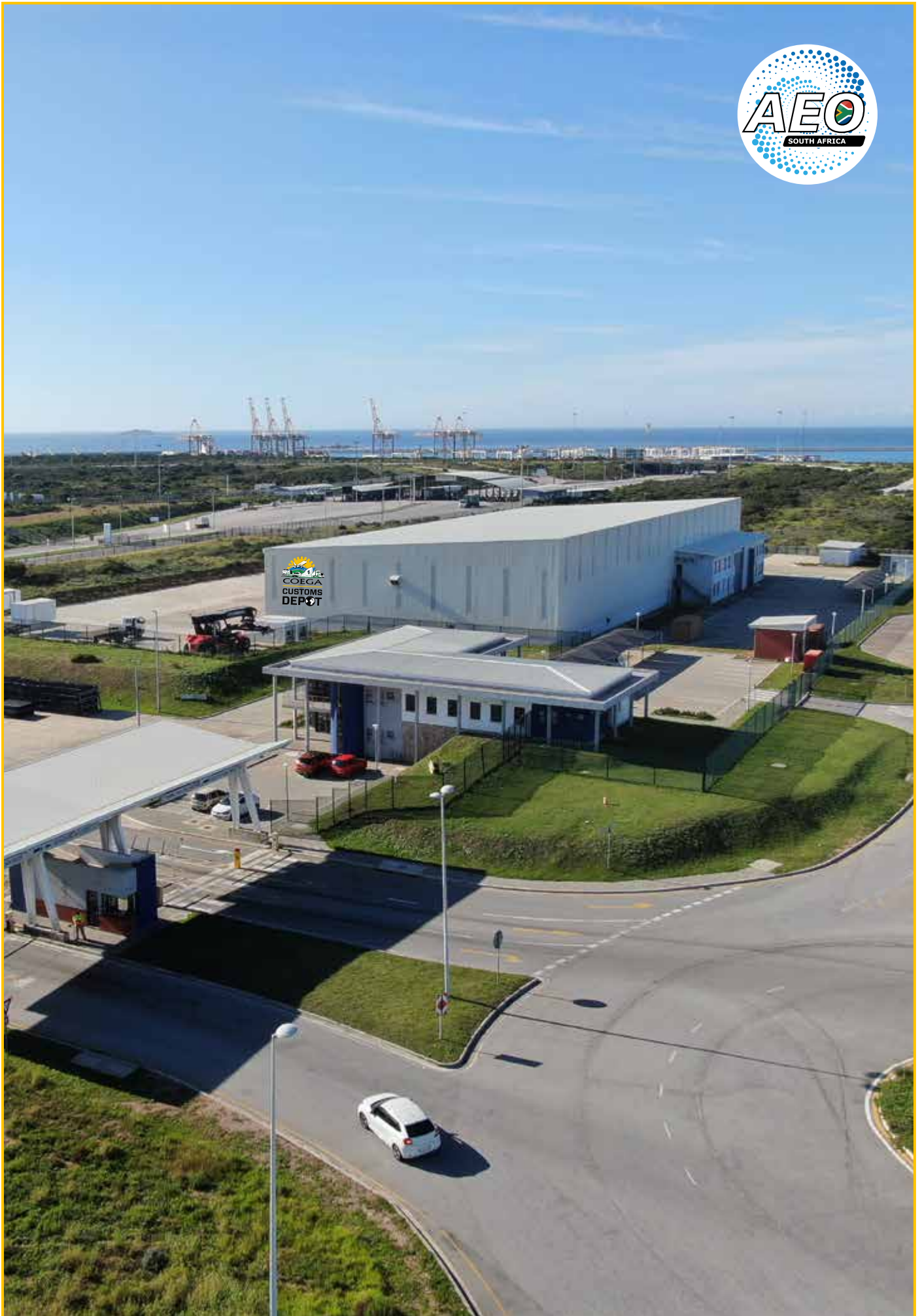
Coega CCA entrance, One-Stop-Shop Building and Customs Depot Warehouse conveniently situated in Zone I of the Coega Special Economic Zone, Gqeberha.
