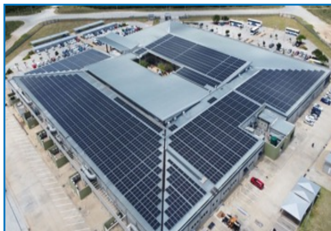
Business Process Outsourcing (BPO) Park, Coega SEZ, Zone 4.
