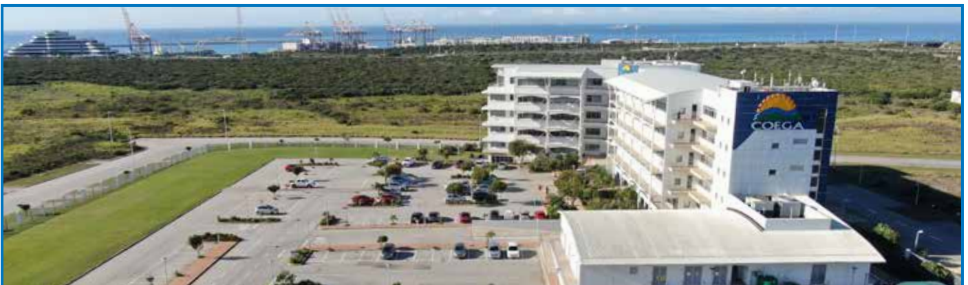
The Head Office of the Coega Development Corporation, with the Port of Ngqura and TNPA Office in the background.
